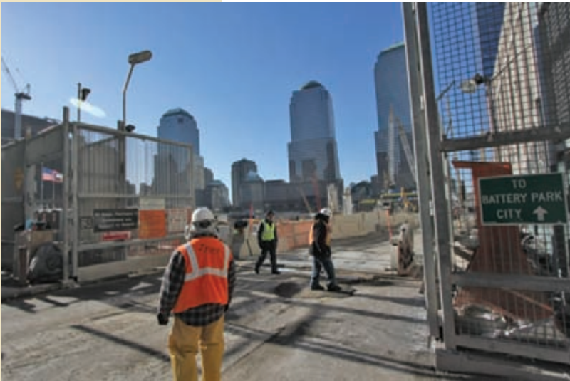
Lower Manhattan, World Trade Center worksite
